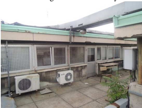
Fig. 11. Roof of FCUB
